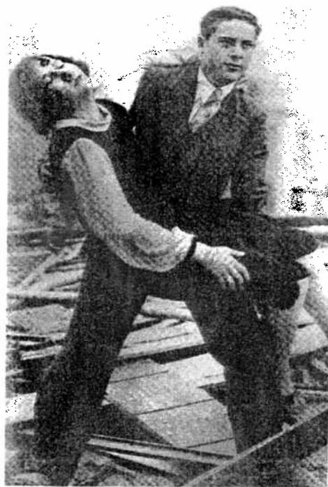
Louis Goldblatt reenacts his rescue of an employee from the Louis Store, which collapsed in 1927 during construction of the five-story Goldblatt Bros. Department Store building addition.
